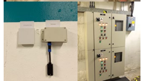
34 sets of IoT temperature and CO sensors (right) and 27 nos of VSD panels for ventilation fans (left) are installed at Three Garden Road's carpark
